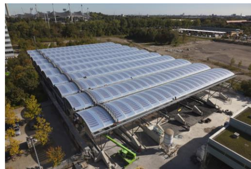
Figure 12 ETFE membrane + flexible thin film PV.
